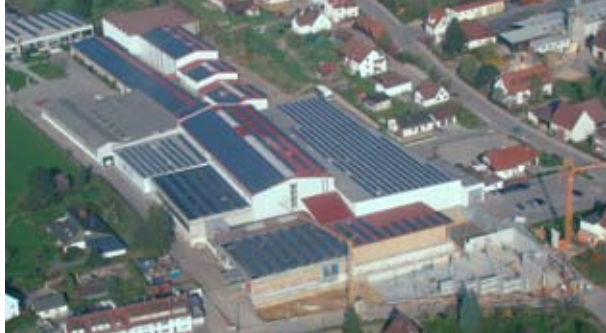
800 kWp power output installed on the hall roofs
