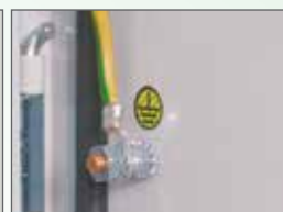
Protective ground connection Bolts on body and door
